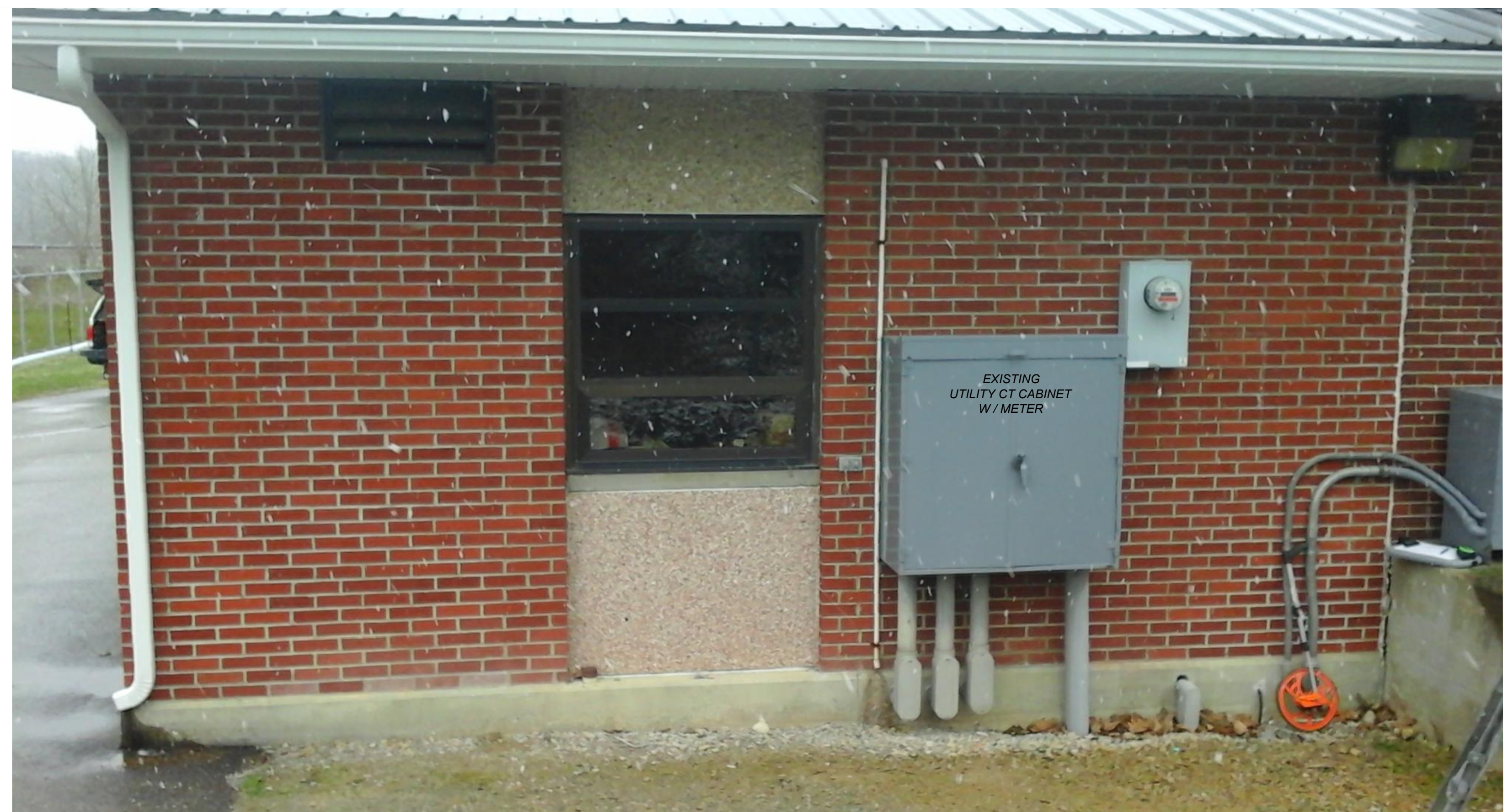
CONTROL BUILDING EXTERIOR - EAST ELEVATION EXISTING CONDITIONS
