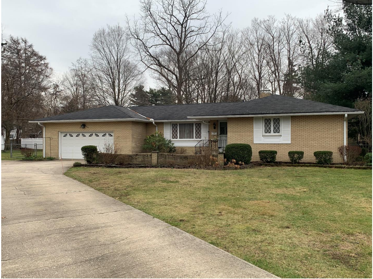
Pre-demolition Photos 7525 Lauren J Drive, Mentor
