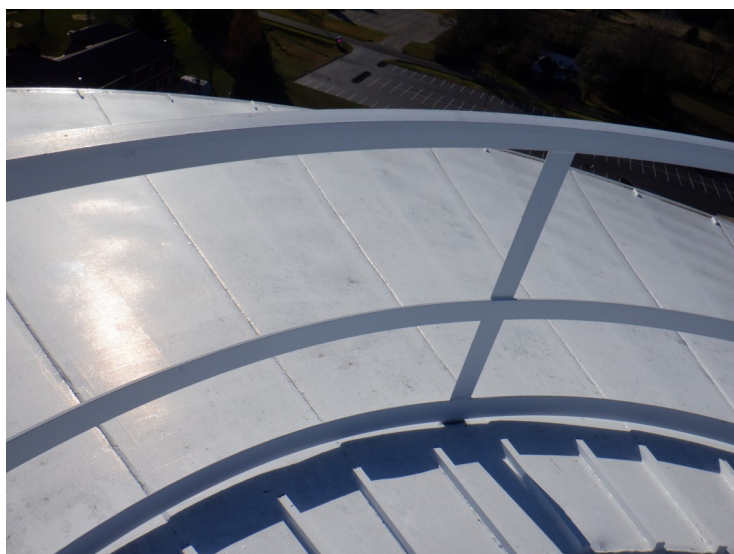
18) The roof handrail is in good condition.
