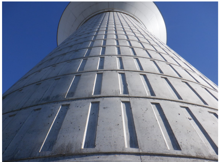
5) The concrete column is in good condition with no deterioration.
