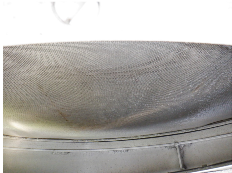
26) The interior roof vent screen is in good condition.
