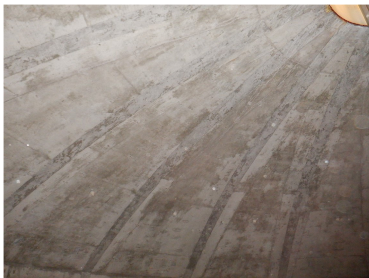
39) There is no concrete deterioration on the domed bottom.
