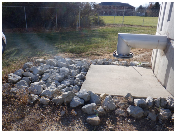
3) The overflow pipe discharges to a concrete splash pad.
