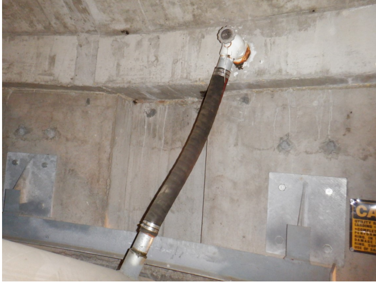
37) The mud valve was not operated during the ROV inspection.
