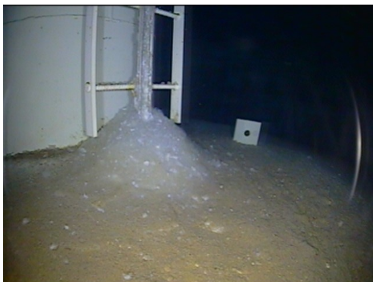
60) The domed bottom was covered in sediment the limited the amount of surface visible with the ROV.
