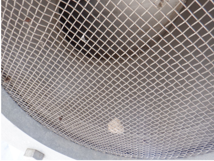
4) The screen at the overflow discharge is intact.
