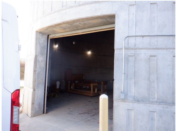
2) The overhead door is in good condition.
