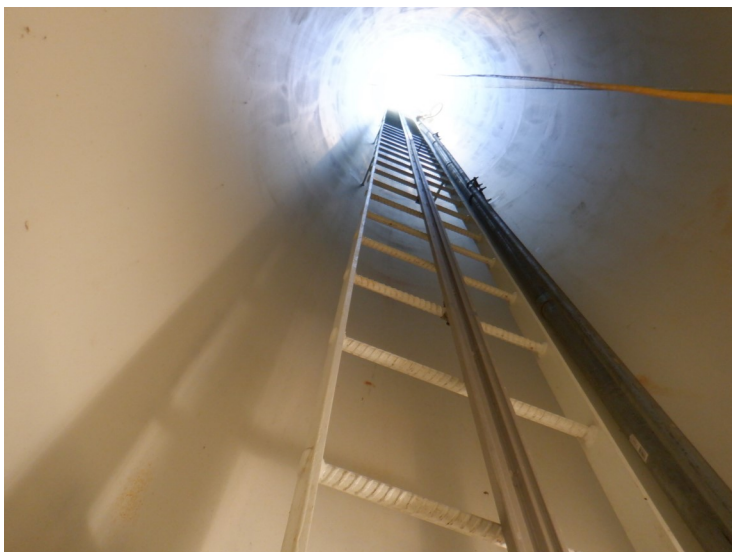
45) The access tube ladder is in good condition. The ladder is equipped with a fall prevention device.
