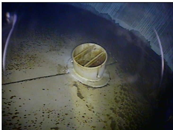
63) There are deflector bars over the fill/draw pipe in the wet interior.
