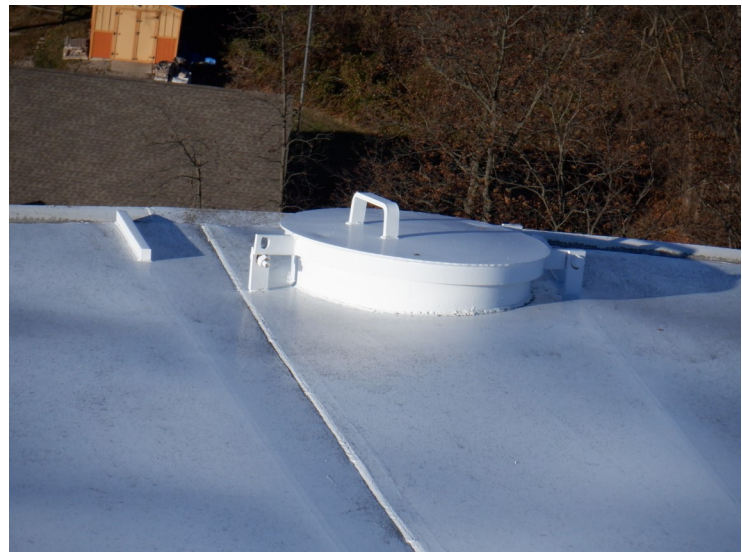
20) The secondary wet interior roof hatch is in good condition.
