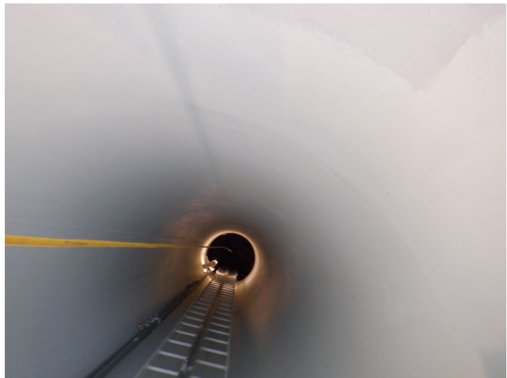
44) The access tube coating is in good condition overall.
