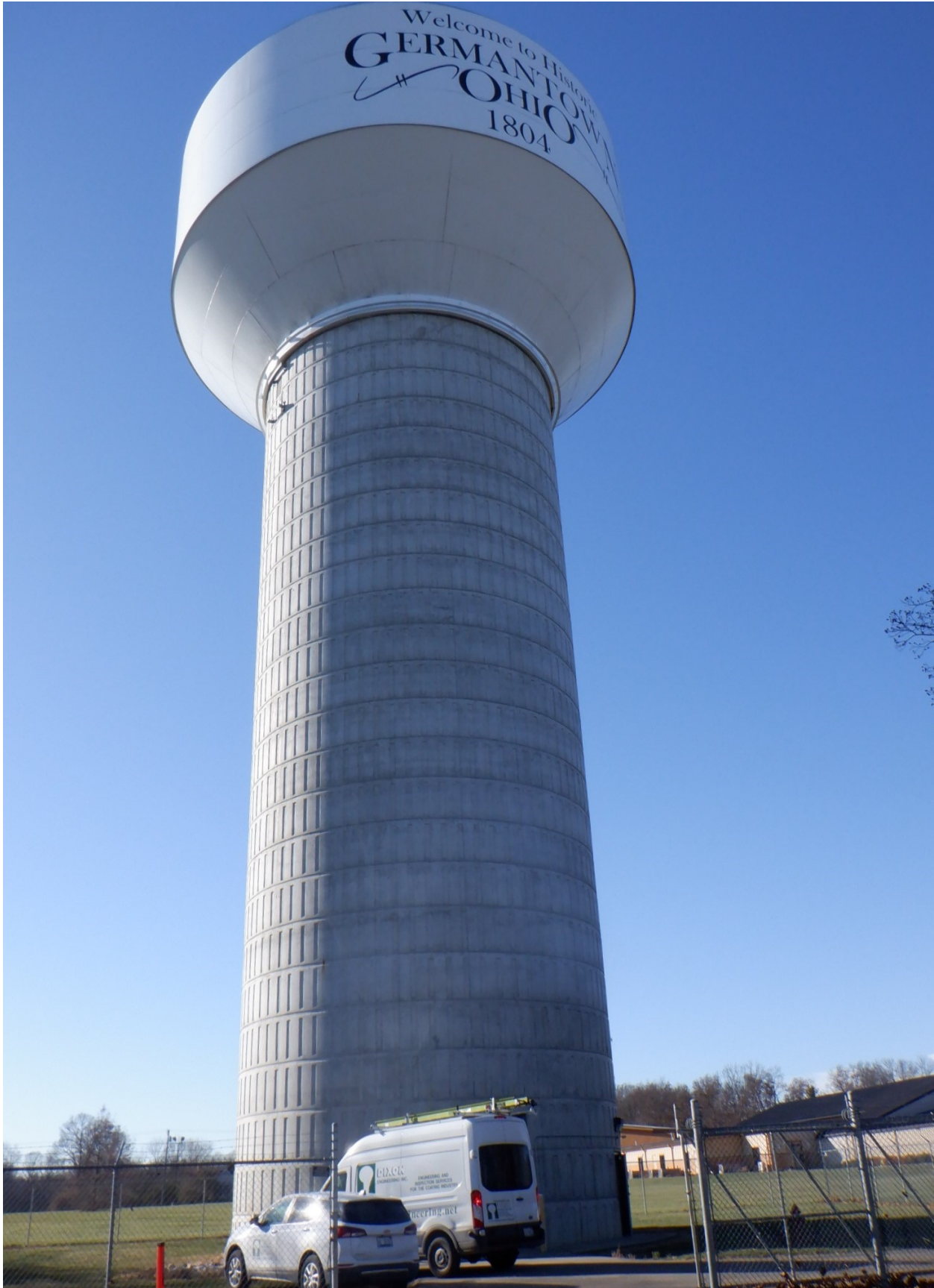
750,000 gallon composite (Route 4) elevated water storage tank owned by the City of Germantown, Ohio.
