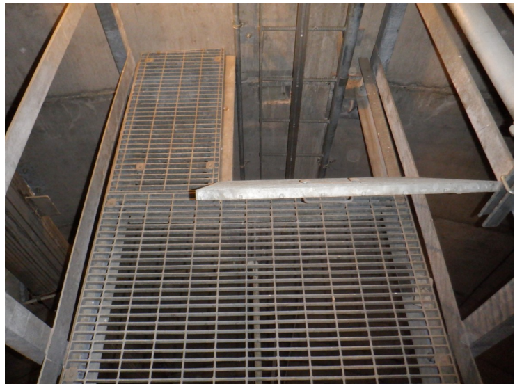
35) The interior platforms are galvanized and in good condition.
