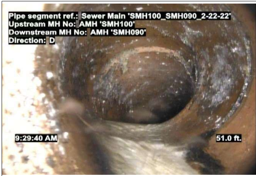
At: 51 ft. 9/. TF - Tap Factory Joint: No
