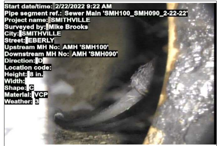
At: 0 ft. AMH - Manhole Joint: No SMH100
