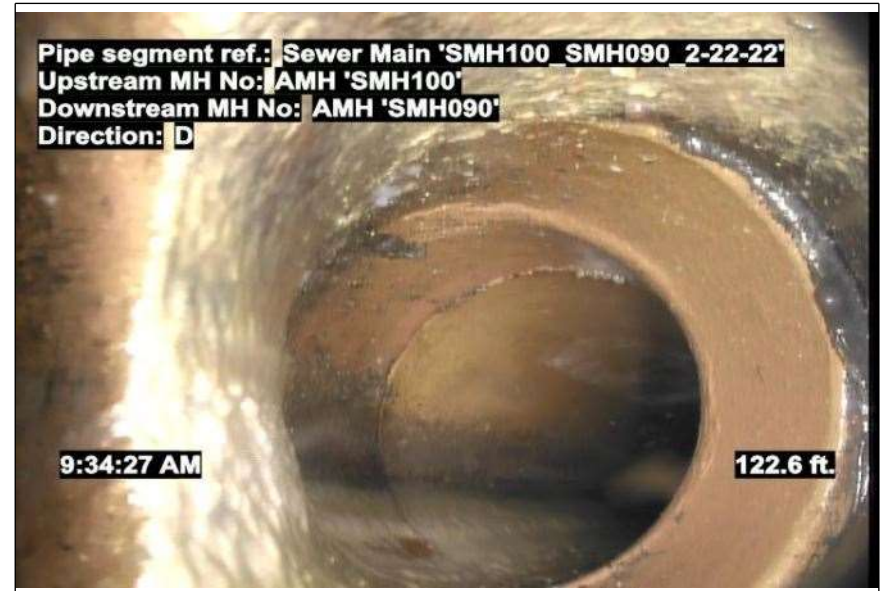
At: 122.6 ft. 12/. TF - Tap Factory Joint: No
