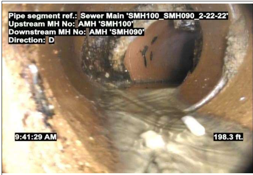
At: 198.3 ft. 9/. TF - Tap Factory Joint: No
