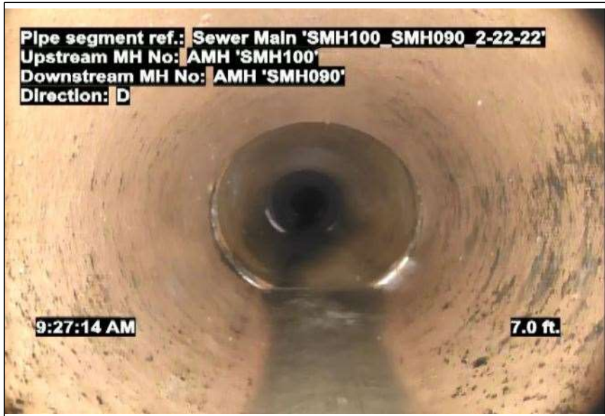
At: 7 ft. MGO - Miscellaneous General Observation Joint: No 7.0FT SET DISTANCE
