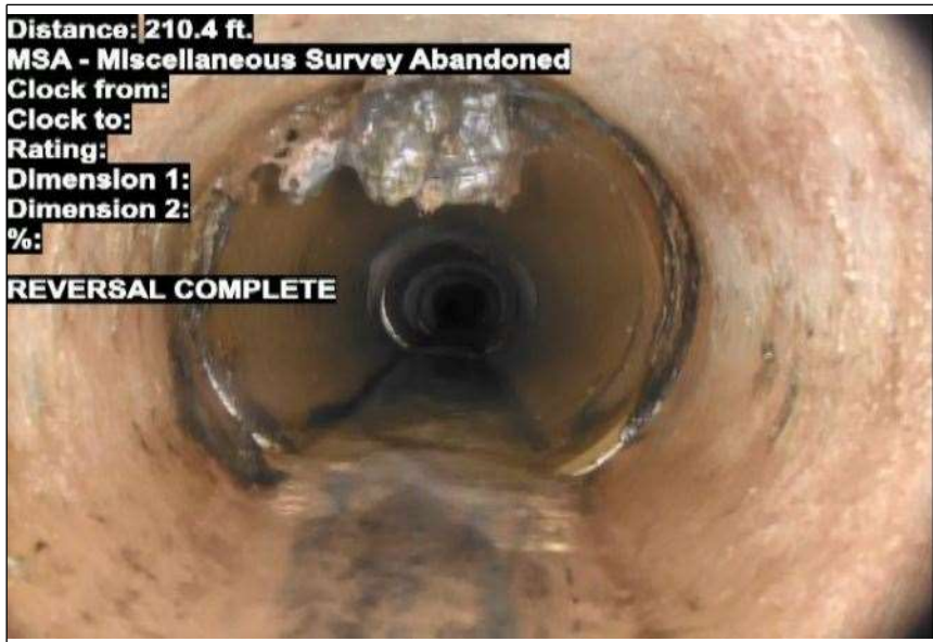
At: 210.4 ft. MSA - Miscellaneous Survey Abandoned Joint: No REVERSAL COMPLETE
