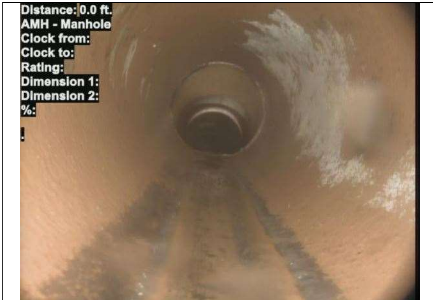
At: 0 ft. AMH - Manhole Joint: No SMH090
