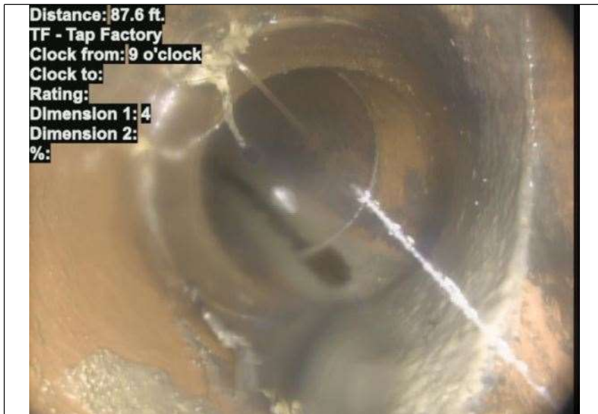
At: 87.6 ft. 9/. TF - Tap Factory Joint: No
