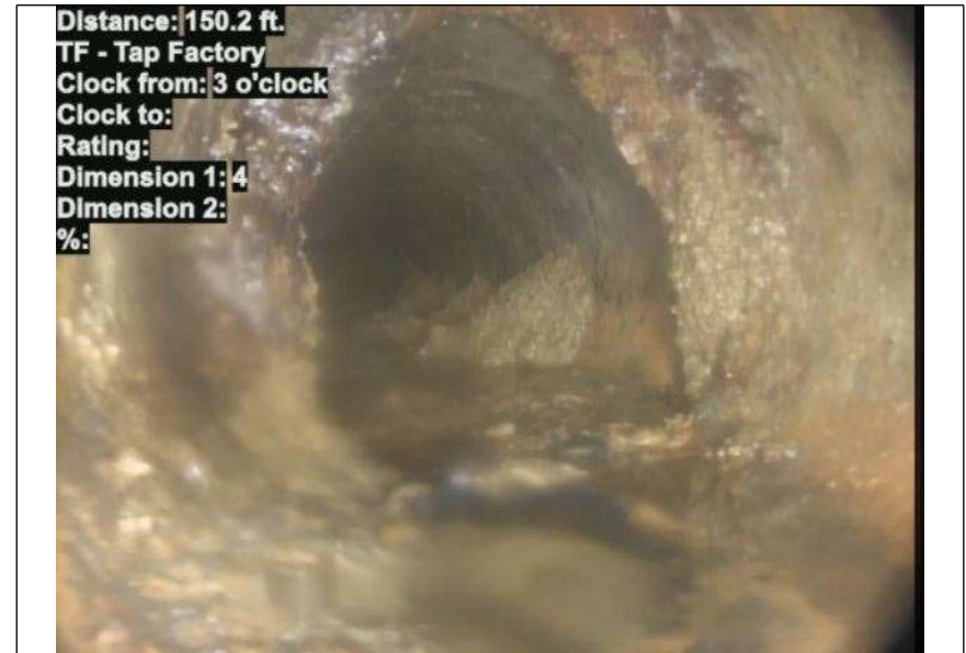
At: 150.2 ft. 3/. TF - Tap Factory Joint: No
