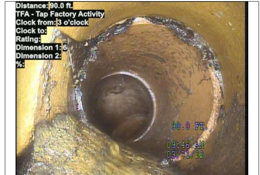
At: 90 ft. 3/. TFA - Tap Factory Activity Joint: No
