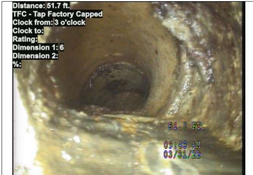
At: 51.7 ft. 3/. TFC - Tap Factory Capped Joint: No
