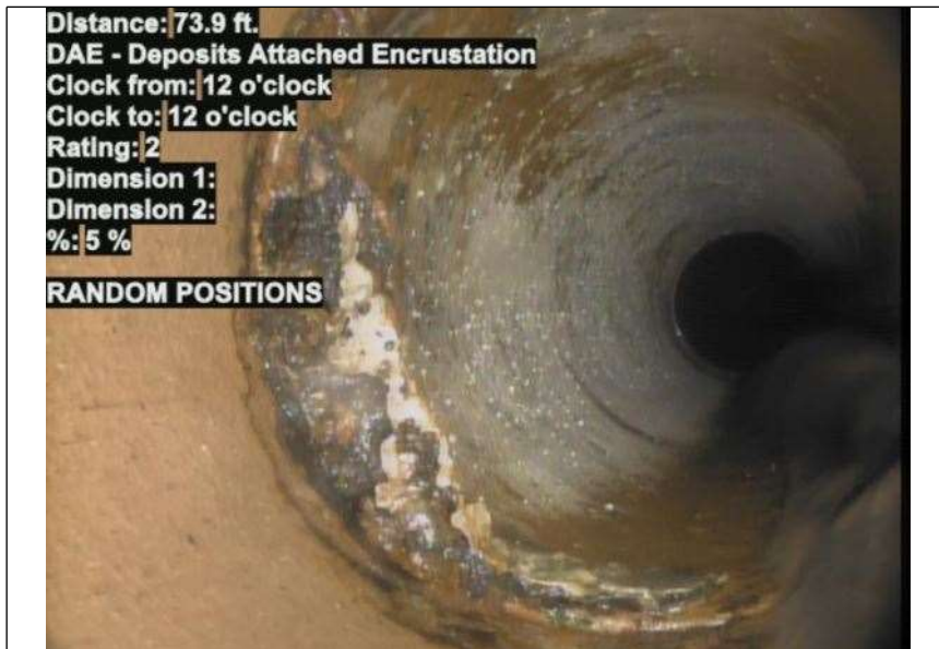
At: 73.9 ft. 7/5 DAE - Deposits Attached Encrustation Joint: No 5 % RANDOM POSITIONS
