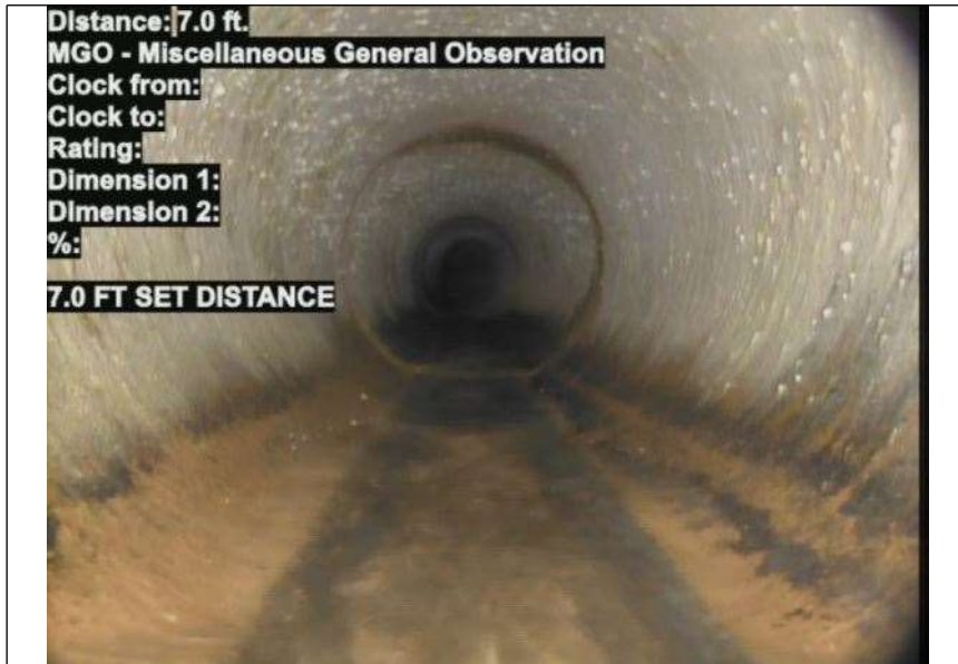
At: 7 ft. MGO - Miscellaneous General Observation Joint: No 7.0 FT SET DISTANCE
