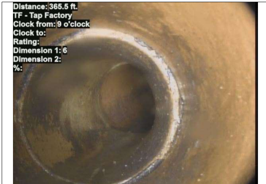
At: 365.5 ft. 9/. TF - Tap Factory Joint: No
