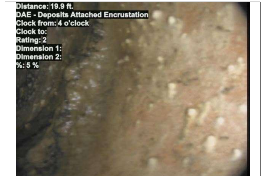
At: 19.9 ft. 4/ DAE - Deposits Attached Encrustation Joint: Yes 5 %
