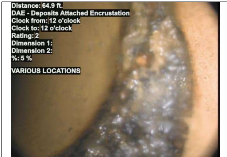
At: 64.9 ft. 7/5 DAE - Deposits Attached Encrustation Joint: No 5 % VARIOUS LOCATIONS
