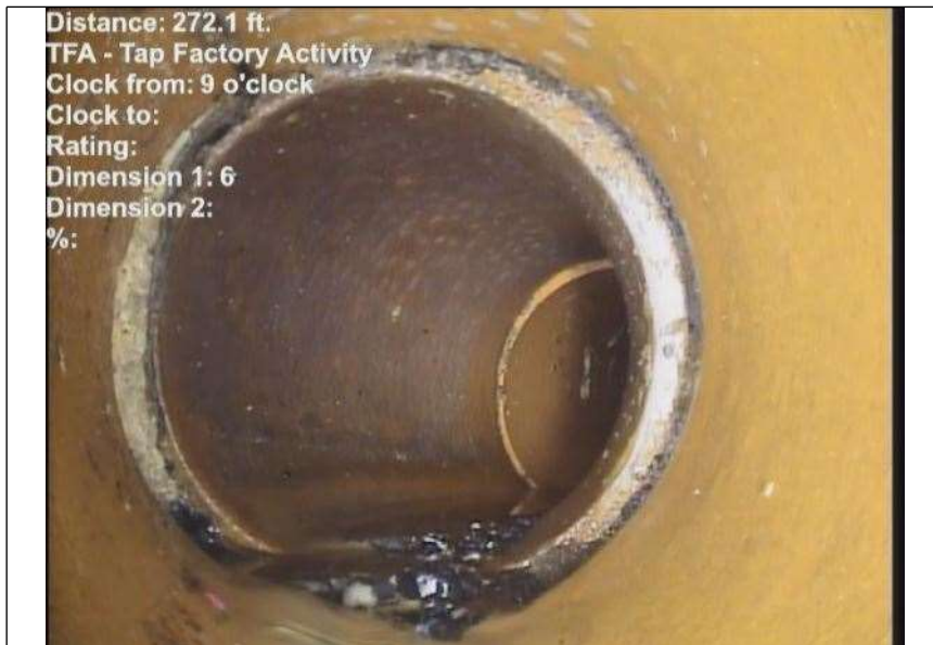
At: 272.1 ft. 9/. TFA - Tap Factory Activity Joint: No
