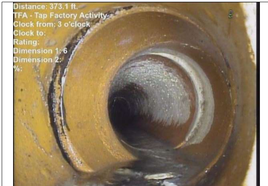
At: 373.1 ft. 3/. TFA - Tap Factory Activity Joint: No
