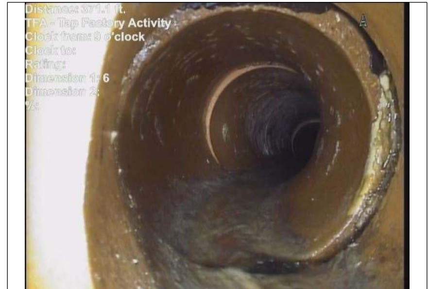
At: 371.1 ft. 9/. TFA - Tap Factory Activity Joint: No
