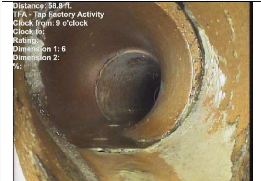
At: 58.8 ft. 9/ TFA - Tap Factory Activity Joint: No
