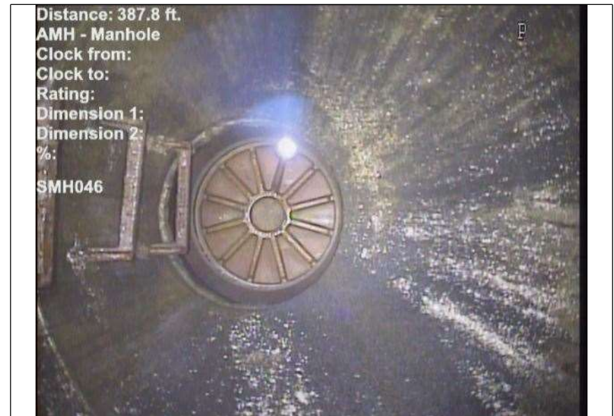
At: 387.8 ft. AMH - Manhole Joint: No SMH046
