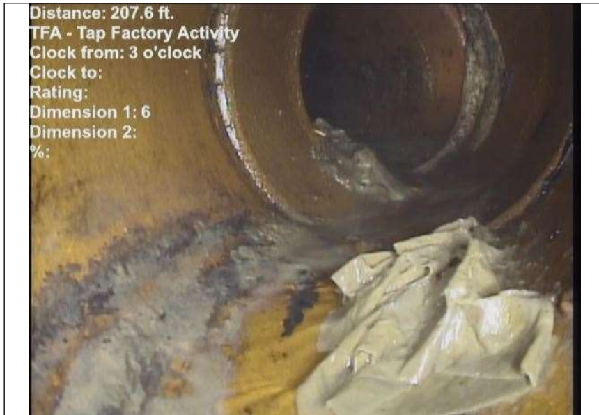
At: 207.6 ft. 3/. TFA - Tap Factory Activity Joint: No
