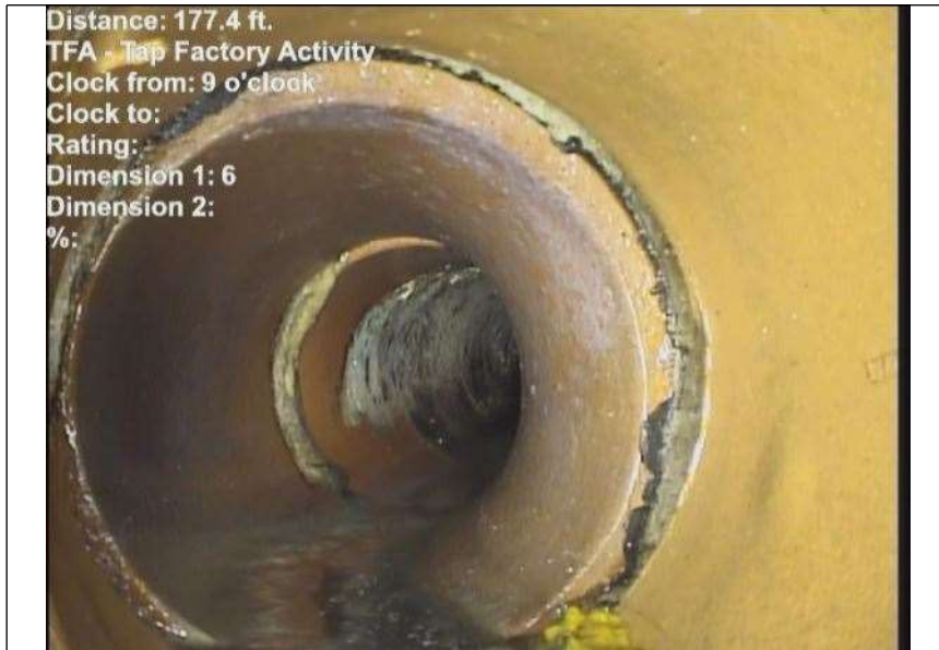
At: 177.4 ft. 9/ TFA - Tap Factory Activity Joint: No
