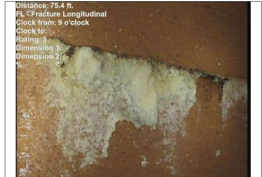
At: 75.4 ft. 9/ FL - Fracture Longitudinal Joint: No
