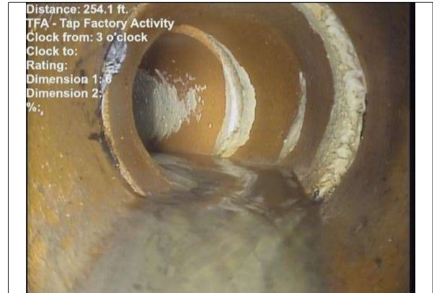
At: 254.1 ft. 3/. TFA - Tap Factory Activity Joint: No
