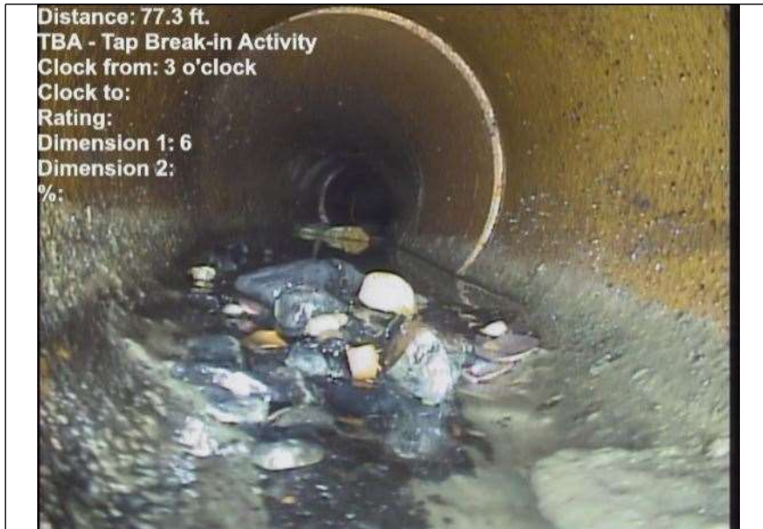
At: 77.3 ft. 3/. TBA - Tap Break-in Activity Joint: No
