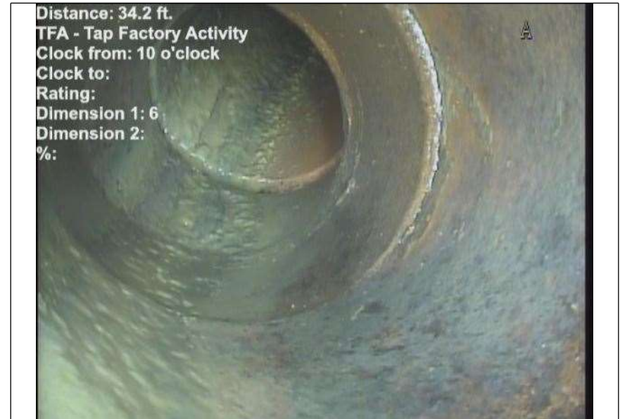
At: 34.2 ft. 10/. TFA - Tap Factory Activity Joint: No
