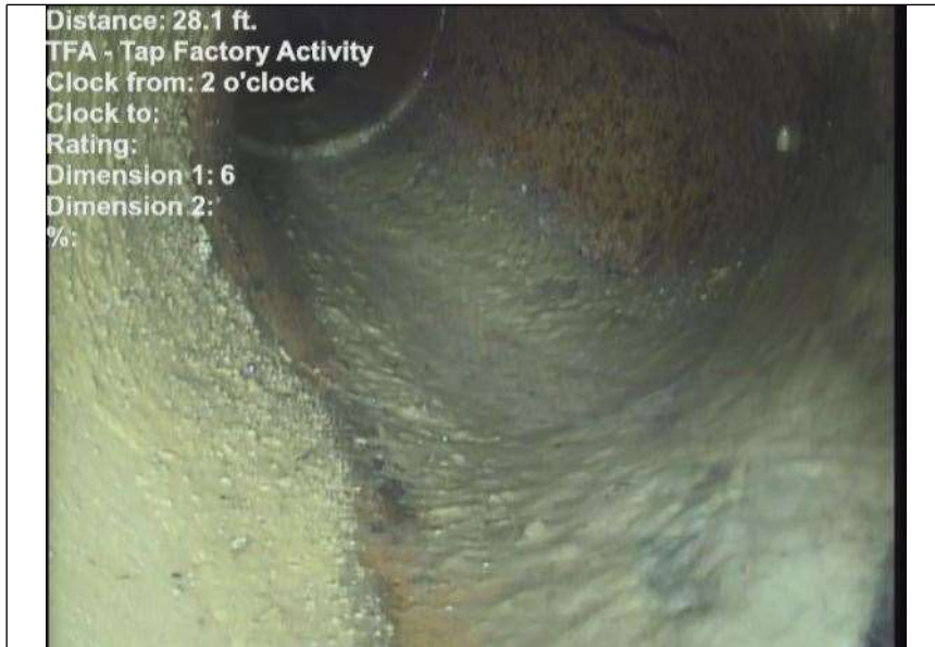
At: 28.1 ft. 2/. TFA - Tap Factory Activity Joint: No
