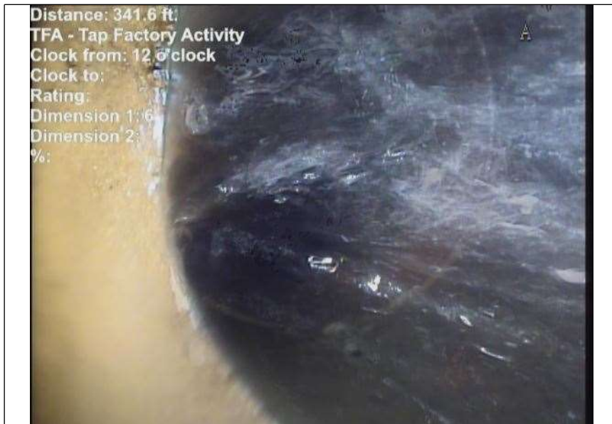
At: 341.6 ft. 12/. TFA - Tap Factory Activity Joint: No
