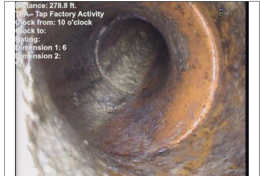
At: 278.8 ft. 10/. TFA - Tap Factory Activity Joint: No
