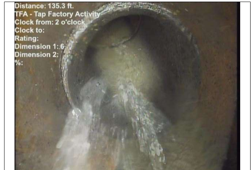
At: 135.3 ft. 2/. TFA - Tap Factory Activity Joint: No
