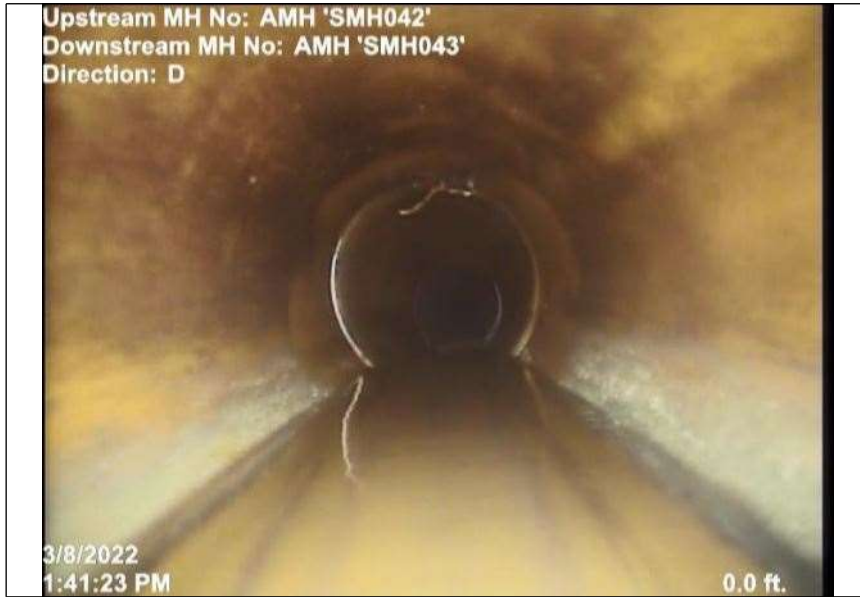
At: 0 ft. MWL - Miscellaneous Water Level Joint: No 5 %
