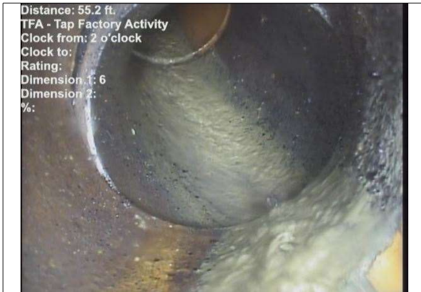
At: 55.2 ft. 2/. TFA - Tap Factory Activity Joint: No
