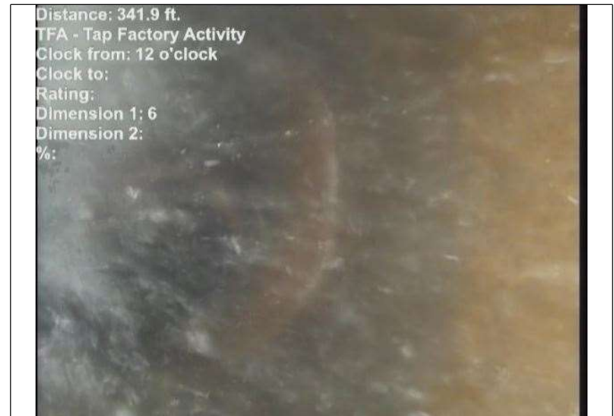
At: 341.9 ft. 12/. TFA - Tap Factory Activity Joint: No
