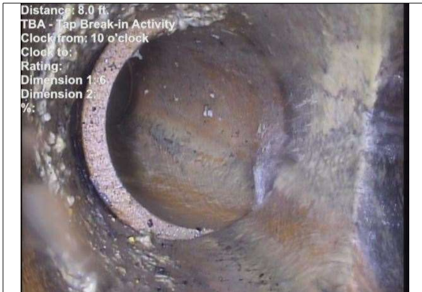
At: 8 ft. 10/ TBA - Tap Break-in Activity Joint: No
