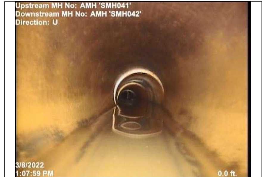
At: 0 ft. MWL - Miscellaneous Water Level Joint: No 5 %
