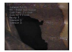
24.0 ft. U HSV Hole Soil Visible 7 / 8
