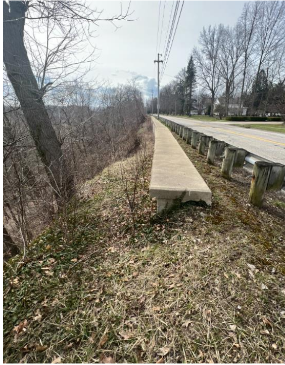
Photo 3: Looking north along river street at adjacent retaining wall
