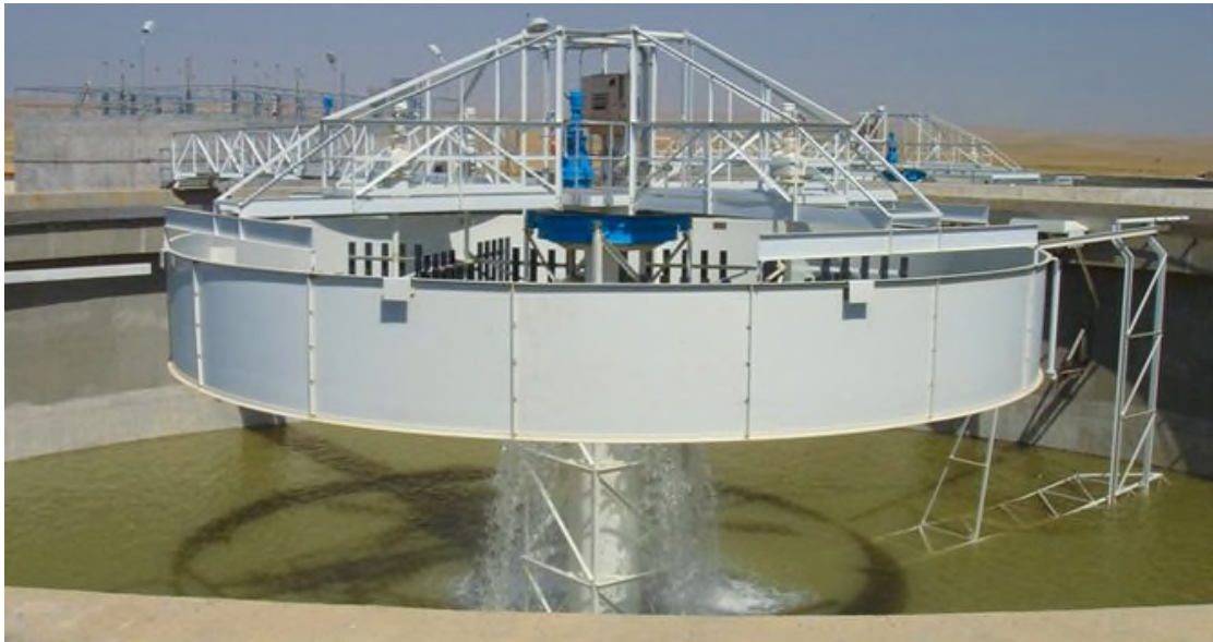
Figure 6-1 – Typical Flocculating Clarifier
