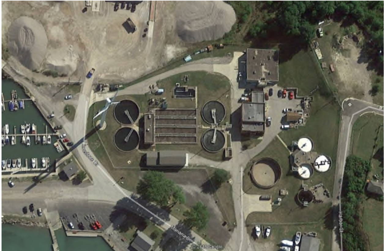
Figure 1.1 – WWTP Aerial Photo
