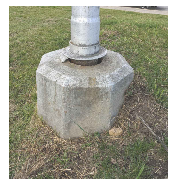
EXISTING FLAGPOLE BASE
