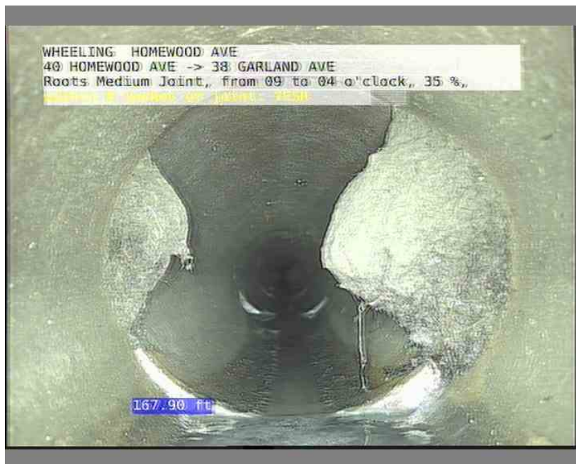
12, 00:12:50, 167.90ft Roots Medium Joint, from 09 to 04 o'clock, 35 %, within 8 inches of joint: YESR
